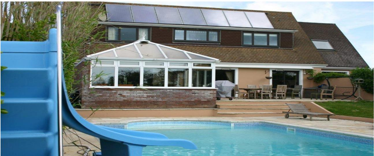
18m<sup>2</sup> of SONNENKRAFT SK500 Flat Plate Solar Collectors were installed, they were laid flat at 35 degrees optimising available roof space and generating greater yields due to the parabolic reflectors and 360° absorbers.
