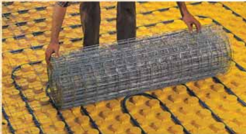
Laying of ANTI-SHRINKAGE MESH
