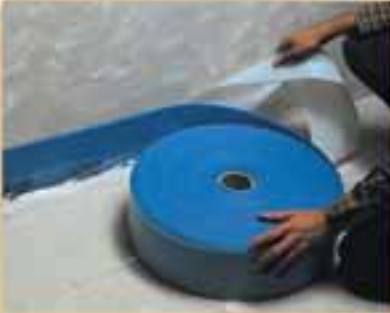
Sticking of the "PLUS" PERIMETRAL FRAME
