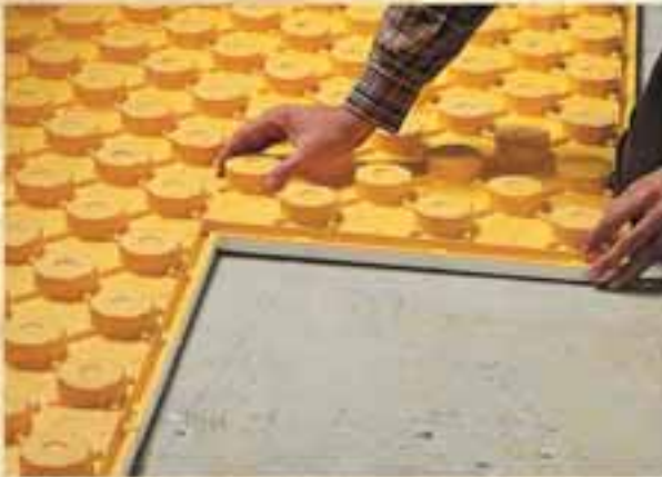
Laying and proper Alignment of "COVER" PANELS
