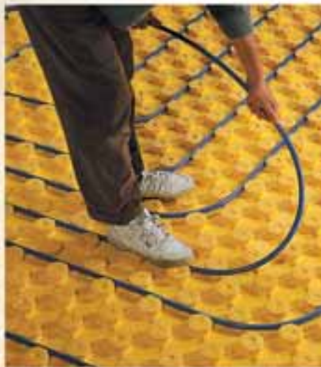
Laying of PE-Xc Pipe
